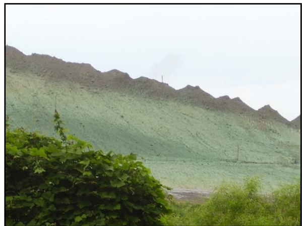
Figure 2 – Wood Based Matrix on Slopes
