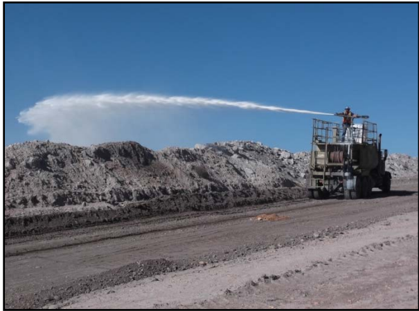
Figure 1 – Application of Polymer Agent
