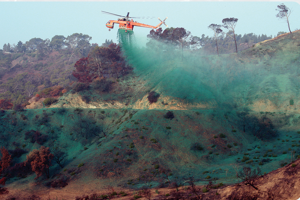
Steep slopes and inaccessible terrain were among the reasons project leaders opted to apply soil stabilization products aerially.
