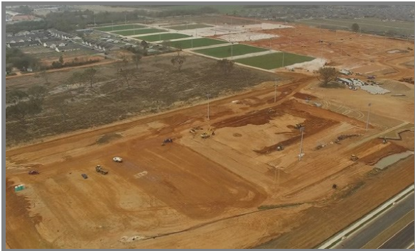
Field construction under way
