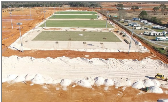
Native sand mixed with 15 percent Profile® Porous Ceramic (PPC) Greens Grade™
