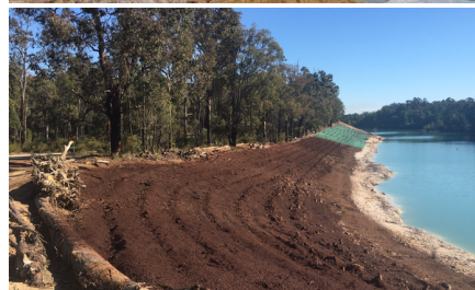
Top: The slope prior to reshaping Bottom: ProGanics applied in the foreground; Flexterra in the background
