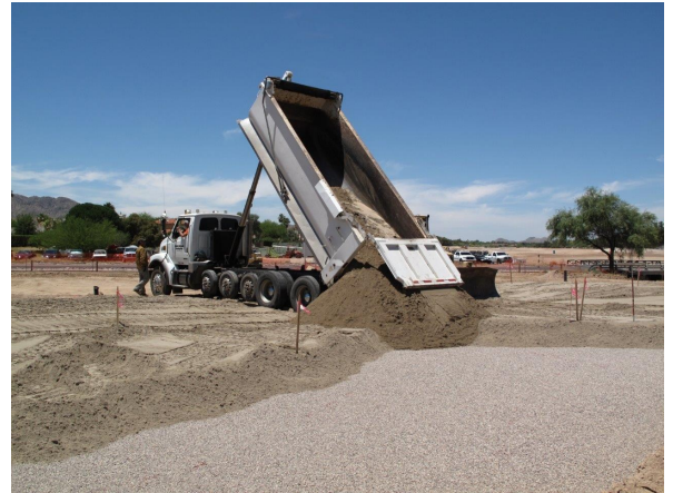
Sand / Profile Blend unloaded for root zone mix installation
