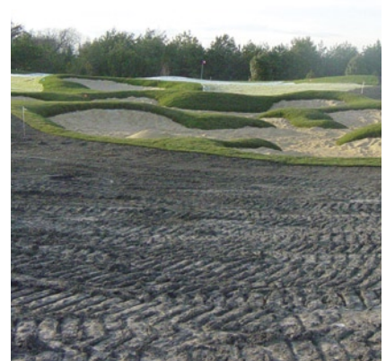
Over 90,000 tons of Profile™ Porous Ceramic-mixed topsoil was created from stockpiled native soil for fairway capping.
