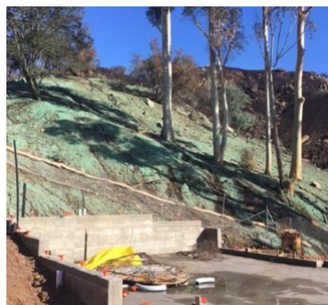
While rain triggered mudslides in the area, Flexterra remained intact
