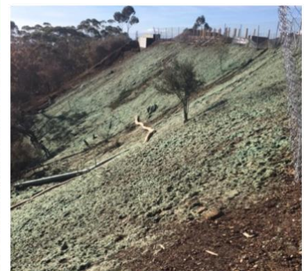
While rain triggered mudslides in the area, Flexterra remained intact
