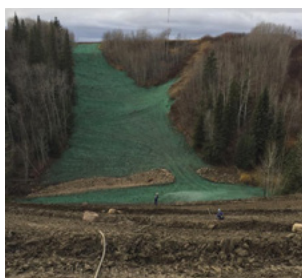
Applying Flexterra® HP-FGM®
