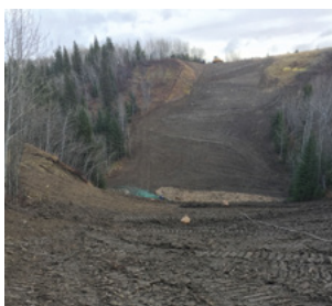
ROW prepped for application
