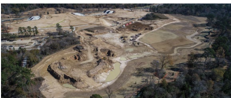
Construction of the Memorial Park Land Bridge
