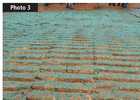
Top looking downslope
