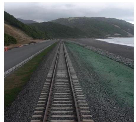
Flexterra application along the road and railways
