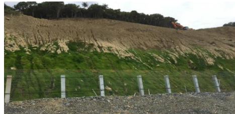
Top: Immediately after the earthquake Bottom: Vegetation fully established on hydroseeded portion of slope 2 months after application
