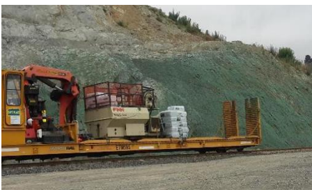
Applying Flexterra to the steep slopes
