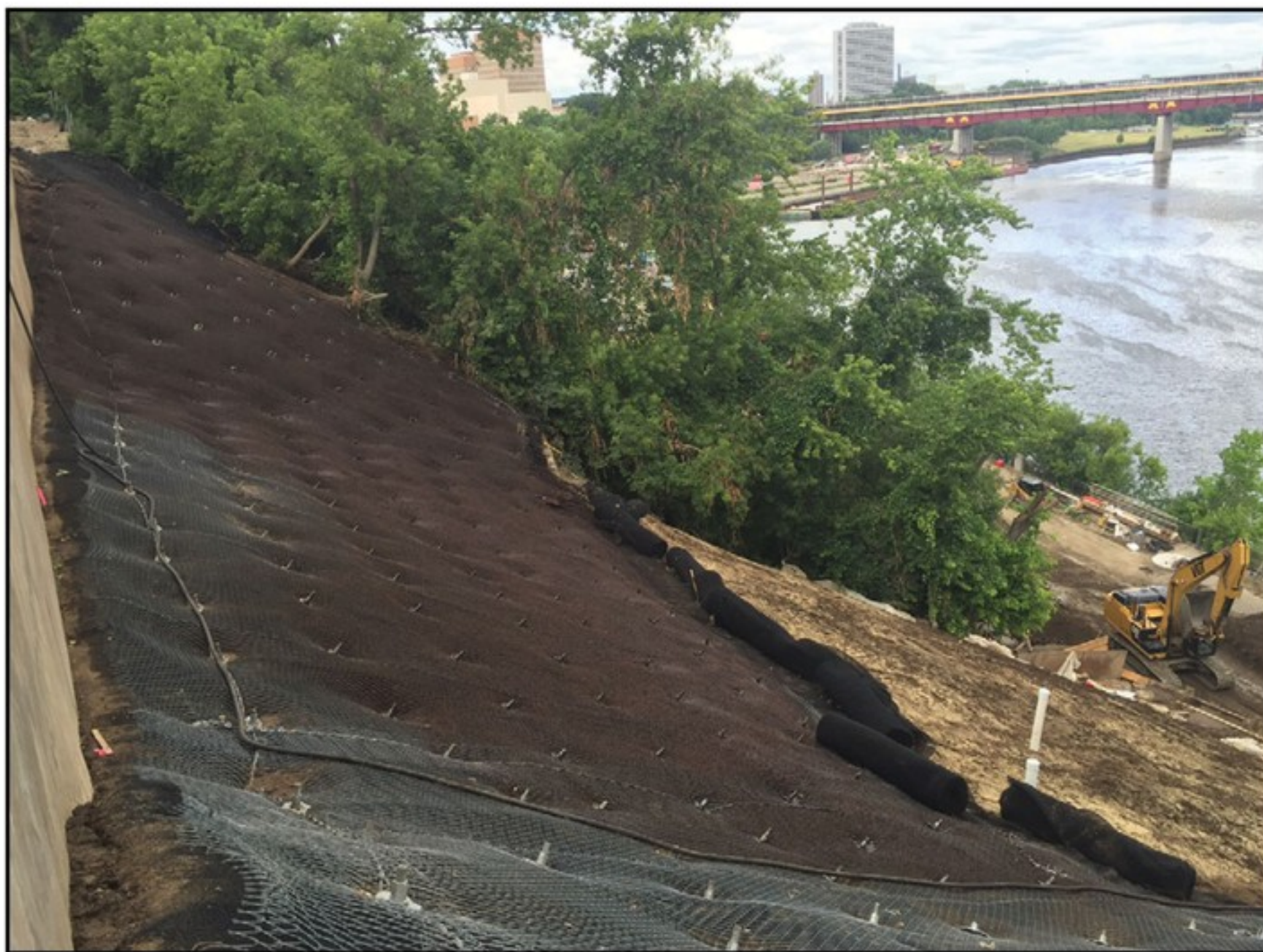
An erosion control design plan was put into place that would address the temporary needs of the slope and maybe more importantly, the long term sustainability of vegetation on the slope.
