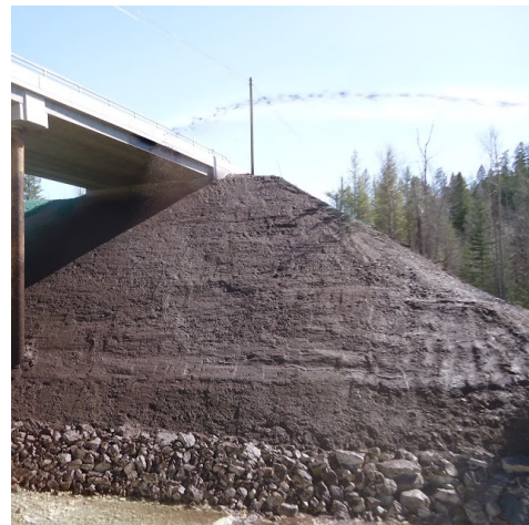
ProGanics installation in March 2016
