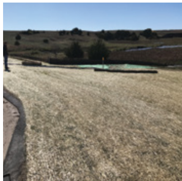
Erosion control installation
