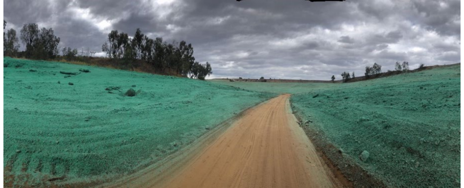
ProMatrix Engineered Fiber Matrix is applied to the site on top of the ProGanics Biotic Soil Media
