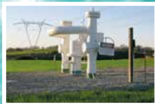
Victory in Vicksburg The MEP Pipeline Project
