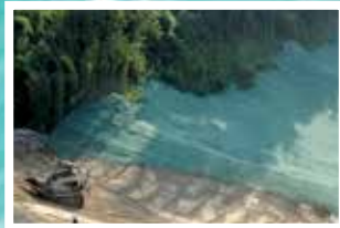
Thirty-mile challenge Rockies Express Pipeline Project
