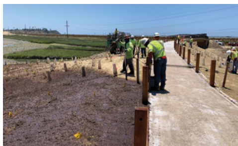
Hydraulically applying ProGanics DUAL in June 2021
