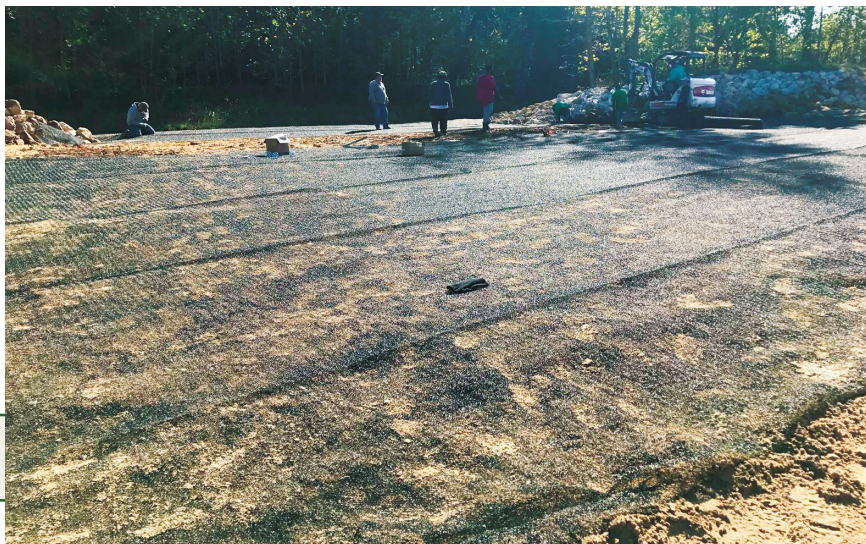
The turf reinforcement mat encourages growth.
