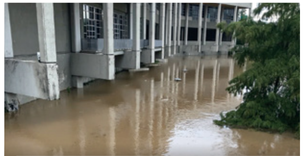
During Tropical Storm Imelda, flooding overtook the site, stressing the reinforced slope and the integrity of the building.
