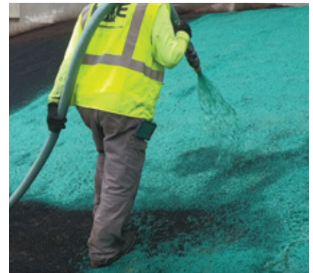
The GreenArmor™ System was capped with Flexterra® HP-FGM® for superior erosion control.
