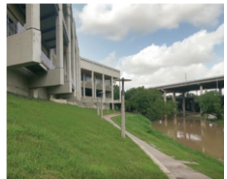
Three months after installation, vegetation had filled in on the slope and was thriving. Construction EcoServices was pleased with the results.
