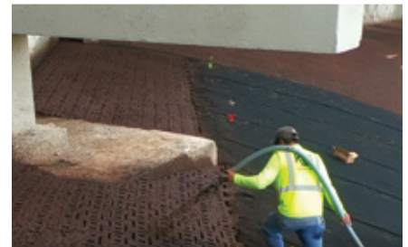
The articulated concrete blocks were hydraulically infilled with ProGanics® BSM™.
