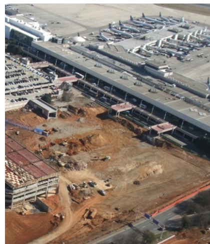
The Charlotte-Douglas Airport required vegetation of more than 25 acres (10 ha), including difficult areas at the end of runways
