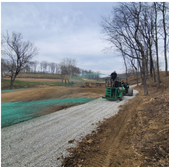
Total coverage of the floodplain with Flexterra® HP-FGM® (March 2023)
