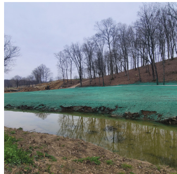
Flexterra® HP-FGM® cures within four hours for immediate erosion protection (March 2023)
